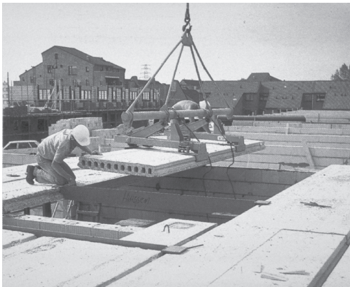
362 Building on the site
