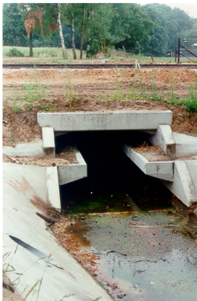
Fig. 315 A prefab culvert with a provision for terrestrial fauna passage (Photo Veenbaas)
