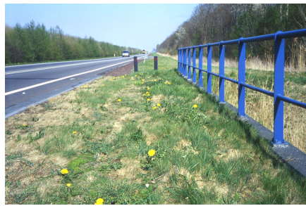
Fig. 314 A viaduct with a vegetated strip connecting existing roadside verges (Photo Bohemen)
