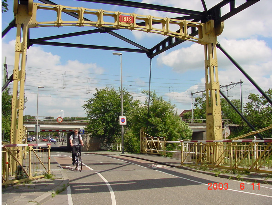
Fig. 503 Neighbourhood street crossing canal and railroad in Utrecht
